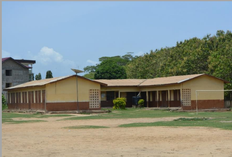
Community School at Kwaprow. This is about 648.3 m from the site.
