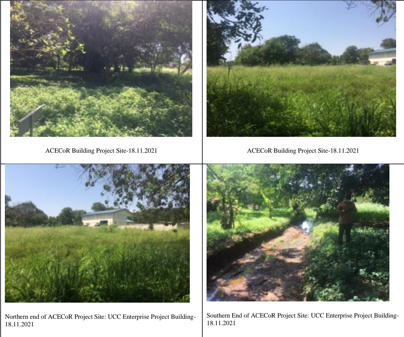
Figure 0-2: Photo Gallery: ACECoR Building Project Site
